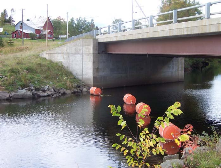
Photo No. 7 – View of the boater restraining barrier upstream of the Route 105 bridge. Note a “Danger Hydro Electric Dam Ahead” sign removed during renovations on the bridge will be re-installed on the bridge guardrails.
