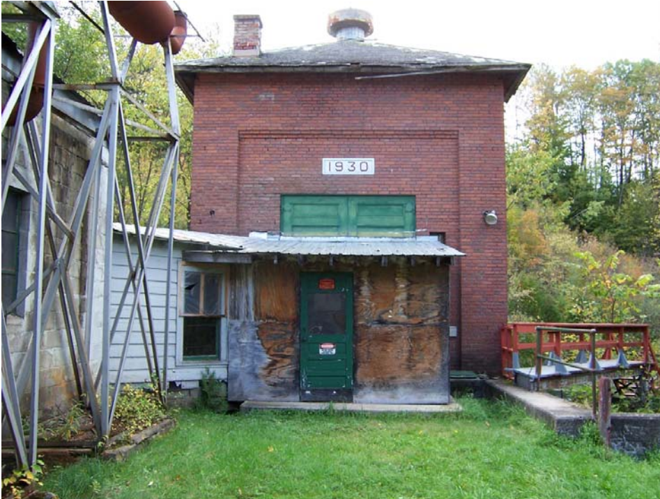
Photo No. 1 – View of the entrance to the powerhouse. This powerhouse was built in 1930 to replace the original hydroelectric powerhouse (circa 1895).
